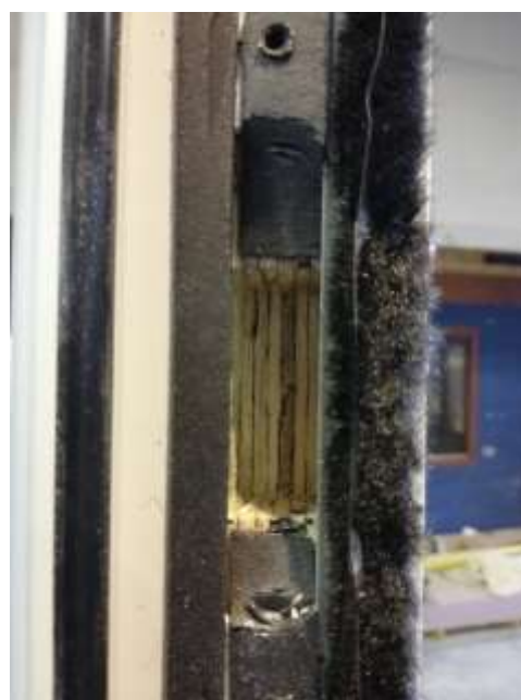
4) Top keep seal interruption (identical to bottom keep)
