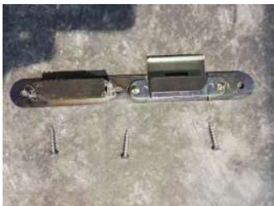
9) Centre latch/lock keep showing intumescent Position
